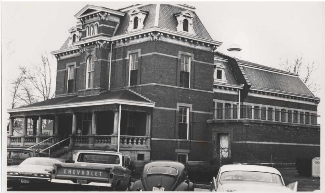
This is the jail with the front porch where the prior picture was taken. This photo was taken around 1961 just a few years prior to demolition.
